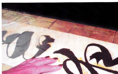
Photo 7: Checking for Trapped Air—Check for potential trapped air by sliding your fingertips lightly across the surface of the film, from center to outer edges, to gently assist air in moving to outer sides and checking for speed bumps.
